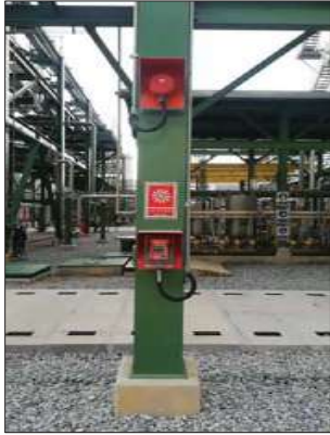
Fire Alarm / Manual call point
